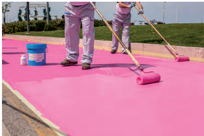
Application of Mapecoat TNS Extreme at Lungomare della Libertà cycle path. Photo: © Mapei
